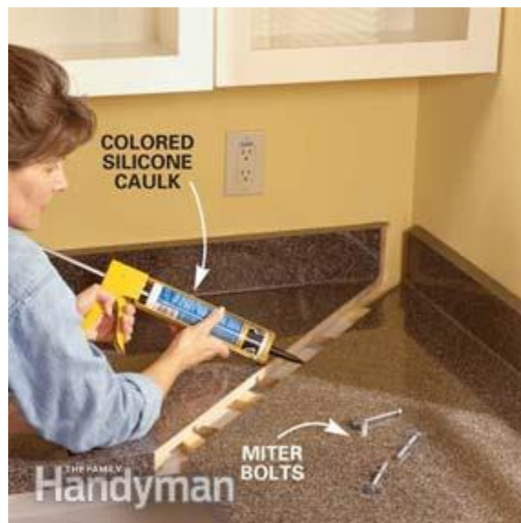
Photo 13: Caulk the miter joint
