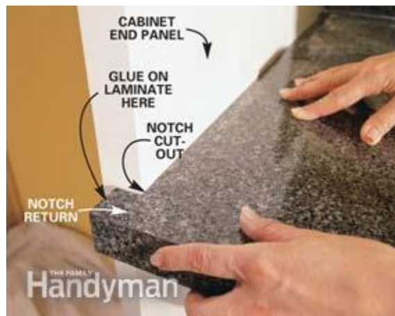
Photo 16: Test fit the countertop notch
