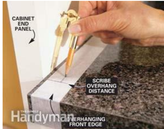
Photo 15: Mark the left side of the countertop
