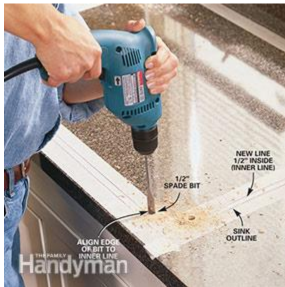
Photo 9: Drill holes inside the template
