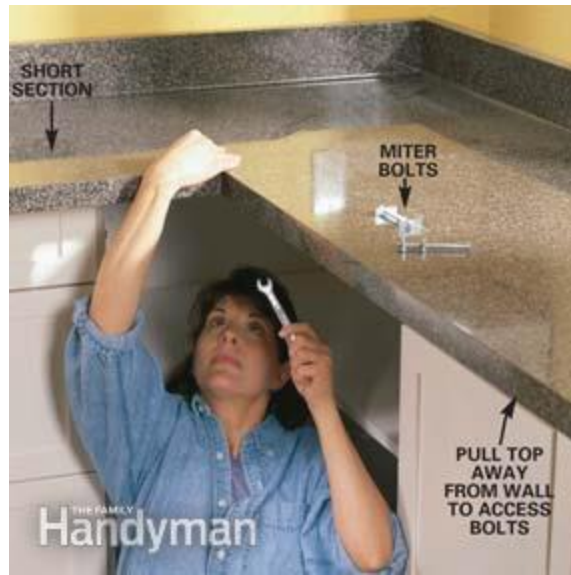
Photo 5: Tighten the miter bolts
